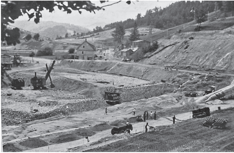
Photo 4 Construction of the dam (private archive)
