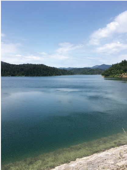
Photo 5 The view from the dam towards Mrzla Vodica (author, 2020)
