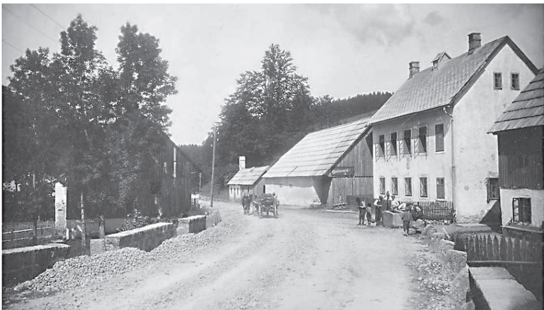
Photo 2 School building in Mrzla Vodica, 1929 (private archive)
